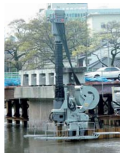
Sheet piling on the water
